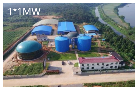
BIOMASS GAS POWER GENERATION PROJECT
