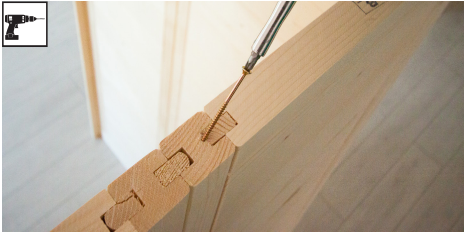
3 mm drill bit, 4 screws 4 x 70 mm
