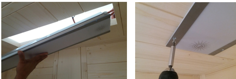
Fig. 50: Installing the colour light
