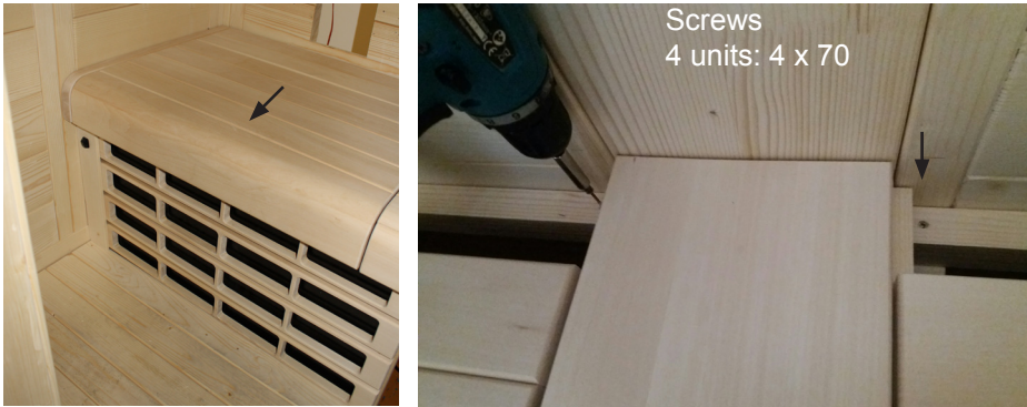
Fig. 51: Attaching the bench
