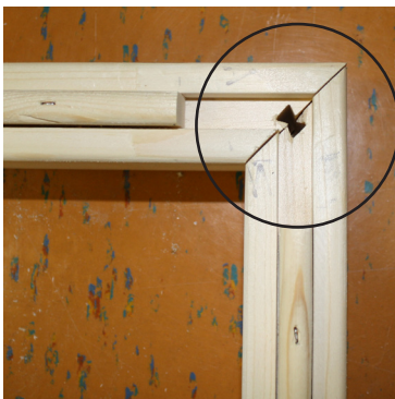
Fig. 2: Connect the floor frame elements
