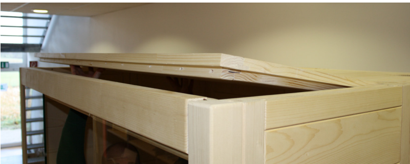
Fig. 18: Installing the roof element in the front
